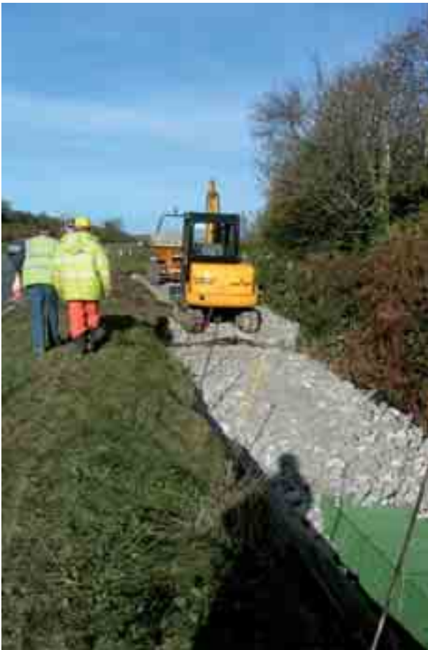
Example of a French drain system being laid
